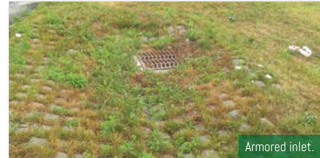
Outlet armored with Flexamat ® , 3 years after installation.
